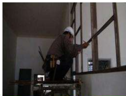
門窗玻璃安裝施作
