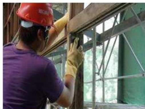
舍房門窗剝漆施作
