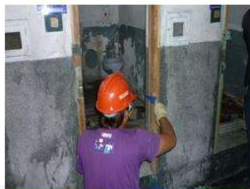
舍房門窗剝漆施作
