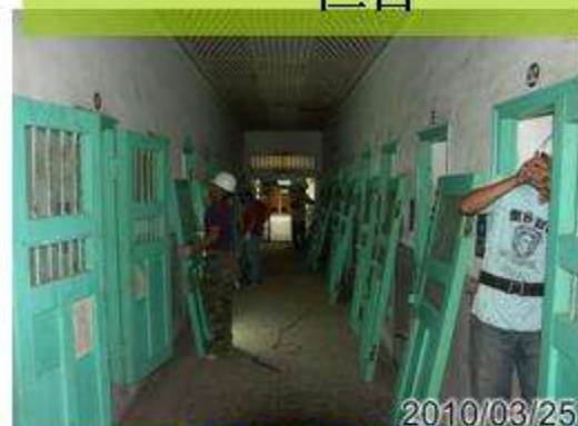
舍房門窗拆卸
