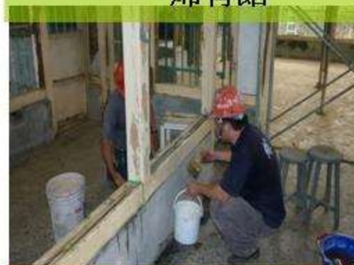
舍房門窗剝漆施作
