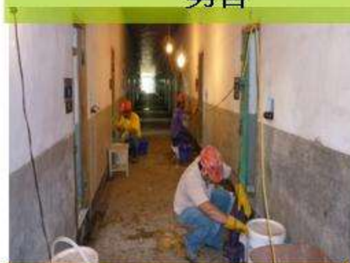
舍房門窗剝漆施作
