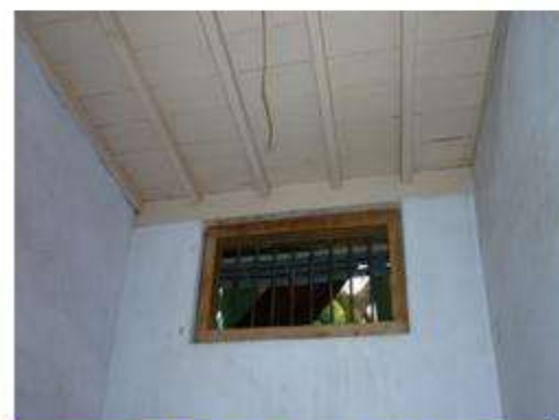
舍房門窗剝漆施作
