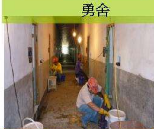
舍房門窗剝漆施作
